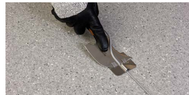
Figure 4a Trimming off the weld top layer (Spatula Trimming Knife)
