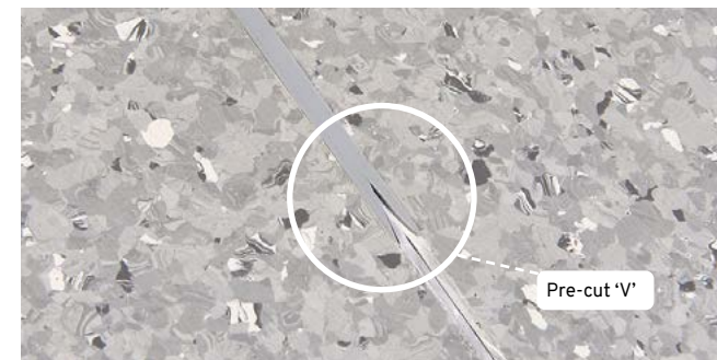
Figure 3 Weld joins
