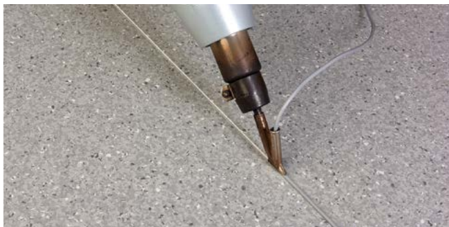
Figure 2 Applying the weld
