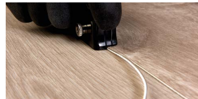
Figure 5 Cutting in the seams
