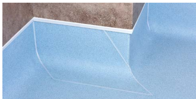
Figure 11 External corners 'wrap around method'
